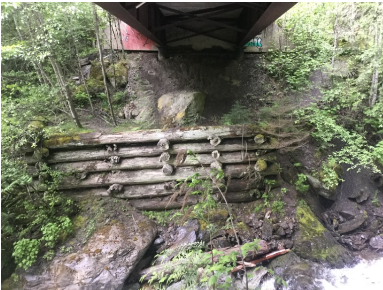
Right Bank Abutment when facing downstream
