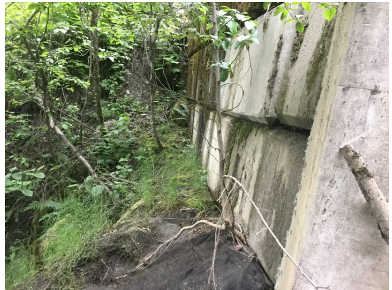
Lock blocks retaining fill at downstream right bank
