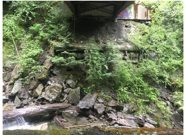
Left Bank Abutment when facing downstream
