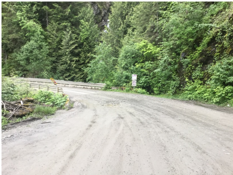
Approach from Left Bank when facing downstream
